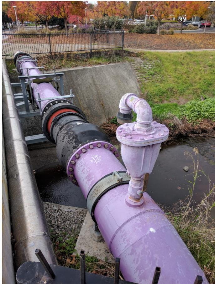
A lavender-colored pipeline carrying nonpotable water in a dual piping system in Mountain View, California. Photo: Grendelkhan, CC BY-SA 3.0
