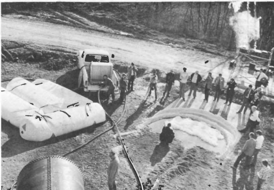
The tank (foreground) leaked liquid which was trapped by plastic foam instant dike. The material was then pumped into plastic container at left.
