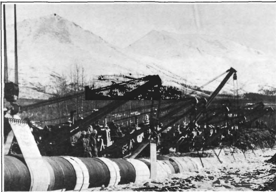
A section of the pipeline is lowered into the ground.
