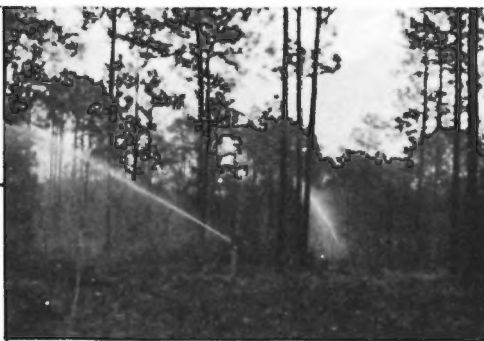
Treated sewage is sprayed onto wooded area at Eglin Air Force Base to avoid polluting a nearby bay used for recreation.
