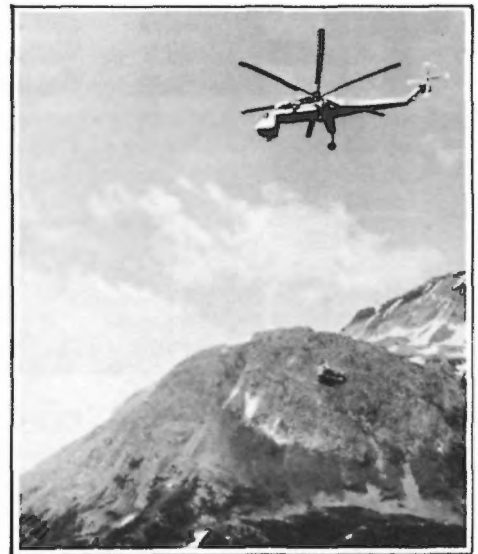
A Sikorsky Skycrane helicopter carries a 10-ton bulldozer to a work location atop the walls of Keystone Canyon, north of Valdez.
