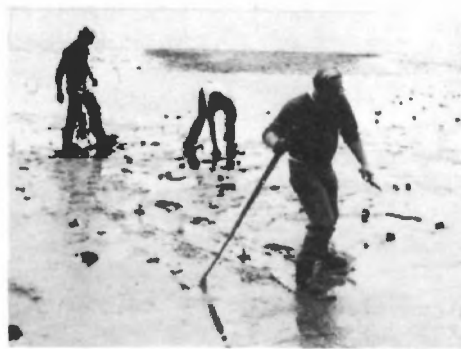
Pots of marsh grass are planted by hand near Quinby, Va., on a tidal flat of dredged material by workmen wearing special shoes to keep from sinking in the mud.
