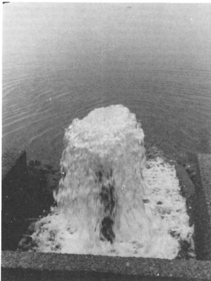
This fountain-like device is an aerator, which pumps lake water up into the air so that oxygen can mix with the water before it spills down a series of concrete steps and returns to the lake.
