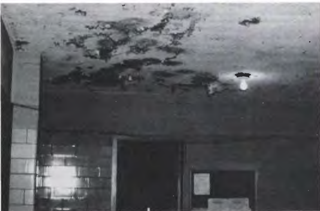
Crumbling ceiling materials could be releasing asbestos particles into the air.
