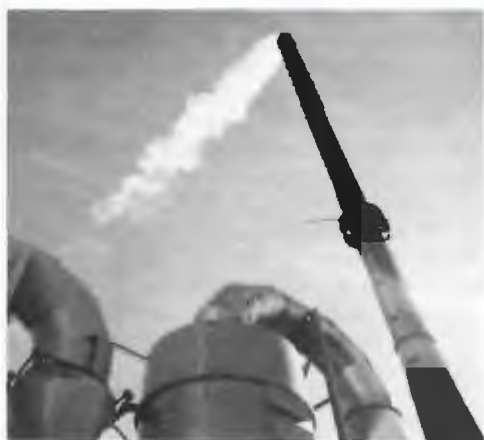
Air pollution control equipment at Chemolite plant at 3M Company in Cottage Grove, Minn.
