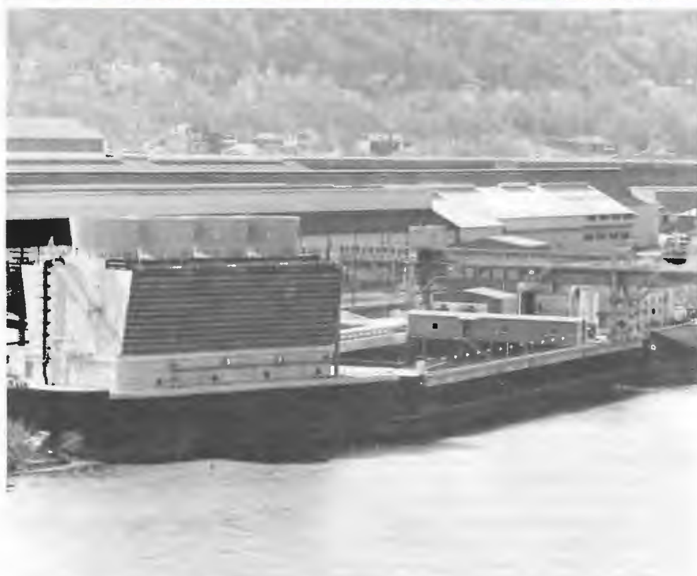
Modern waste treatment facilities at a U.S. Steel plant at the Homestead Works near Pittsburgh.
