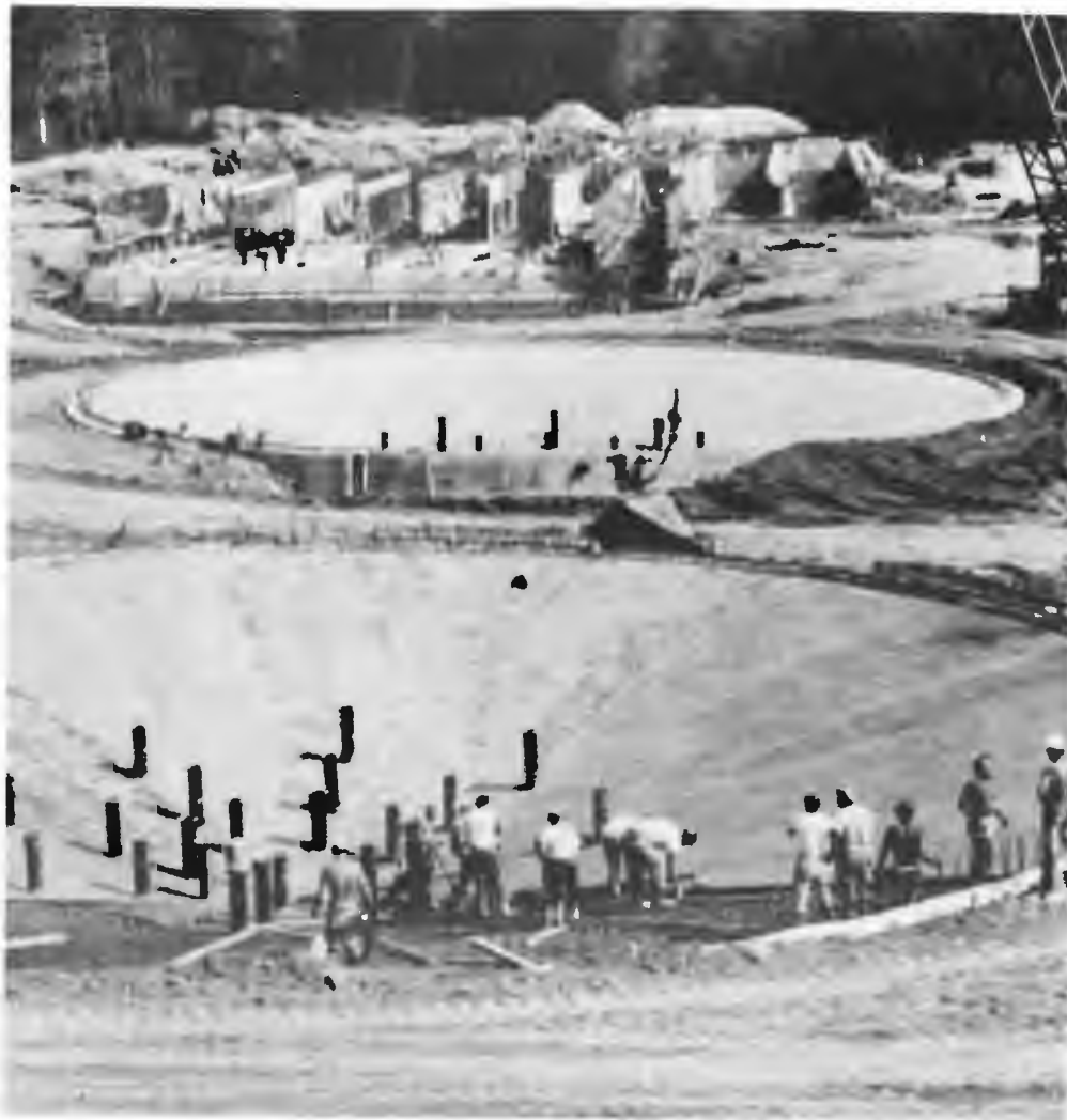
Construction under way on new wastewater treatment plant facilities.
