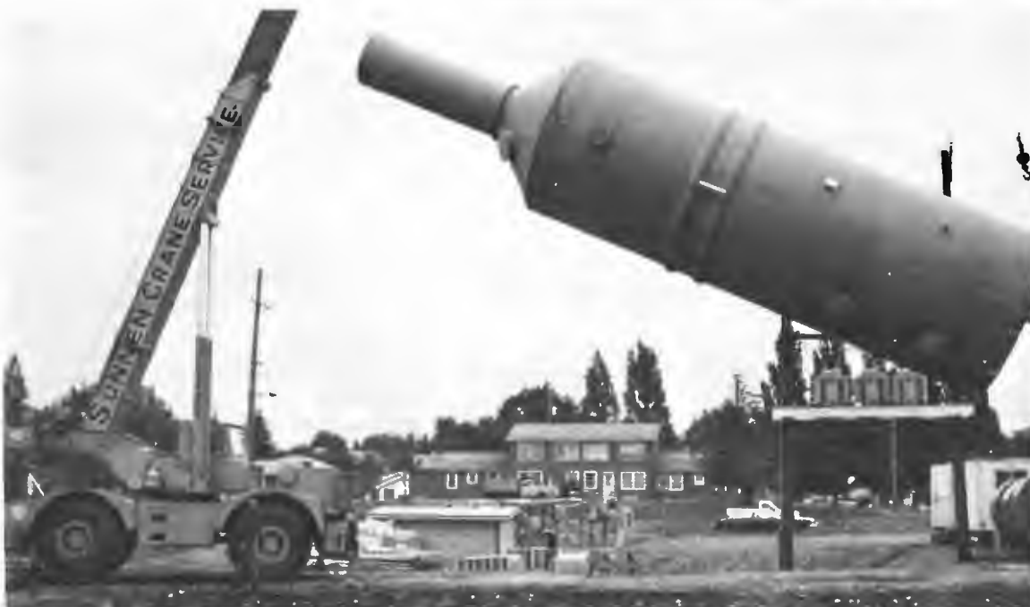
Stripping tower is lifted into place by a crane.
