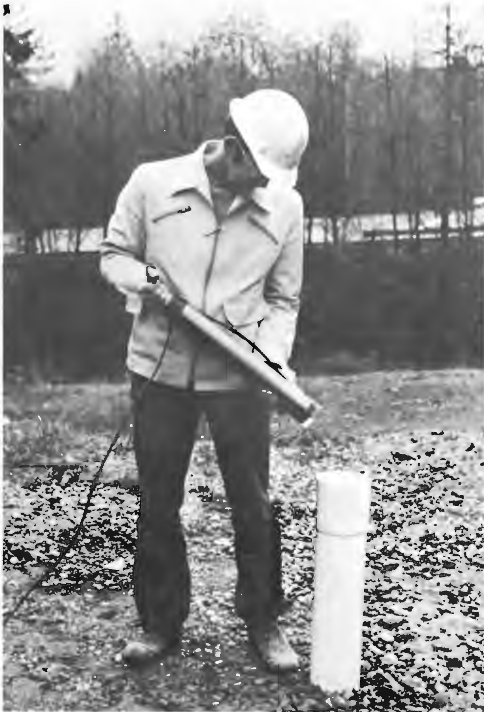
installing a sampling well in a monitoring cell.
