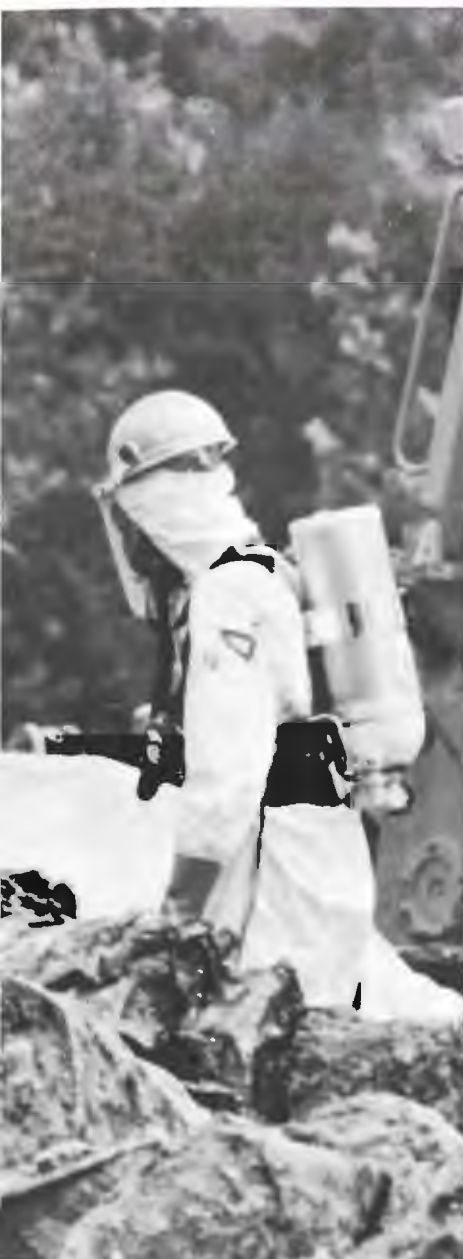
In front of a pile of contaminated soil, workmen cover deteriorated drums of lead-based paints with plastic sheeting. The sheeting will prevent the lead from leaching into the soil during wet weather. A builder preparing the ground for house construction discovered the buried drums in Calverton, Maryland. Concerned about off-site migration of lead, EPA initiated a removal action to dispose of the drums and polluted soil.
