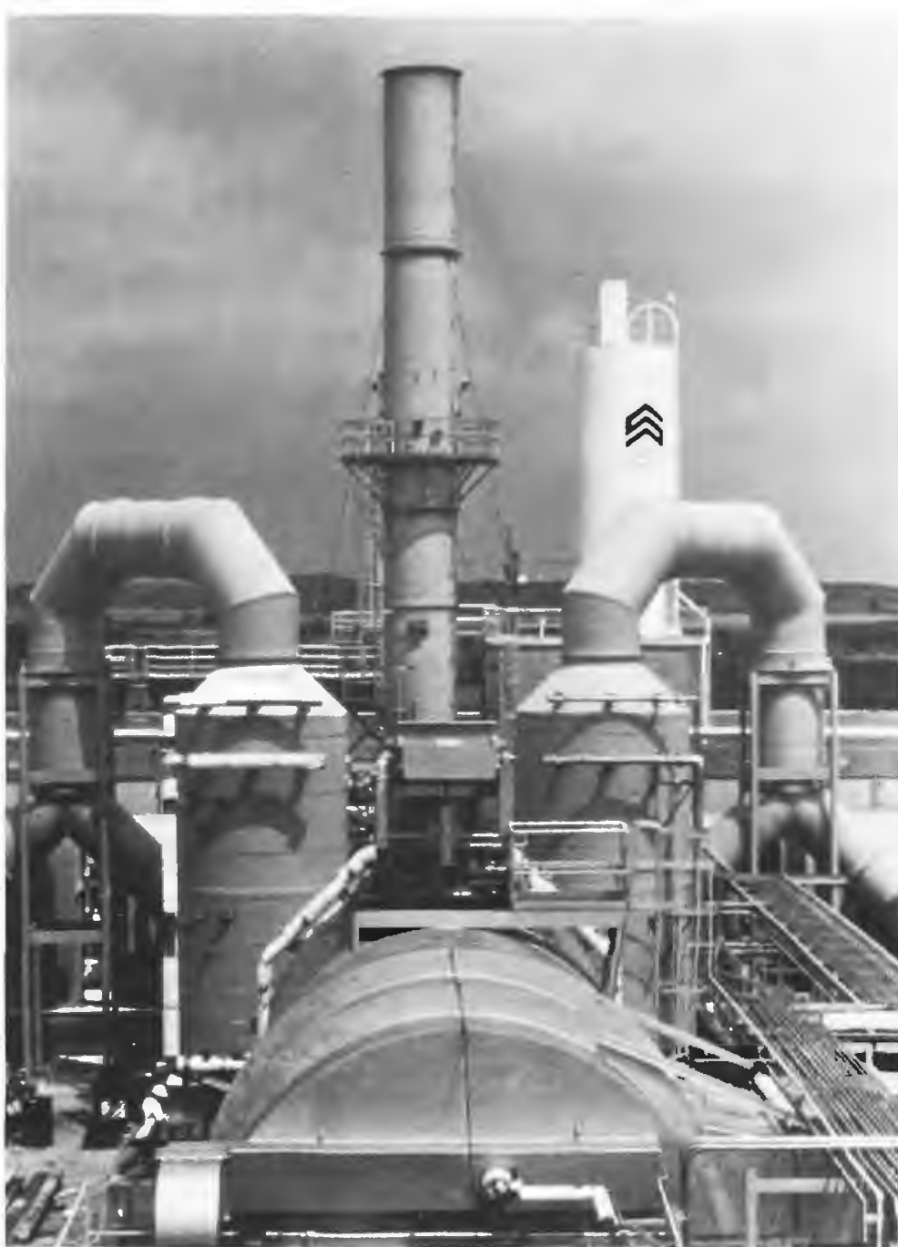
Main combustion chamber of the Chicago incinerator is in the foreground. On either side of it are the two scrubbing towers — a vertical pack scrubber and an ionizing wet scrubber. In the rear is the stack; and, next to that, the lime tower used in the acid neutralization process.
