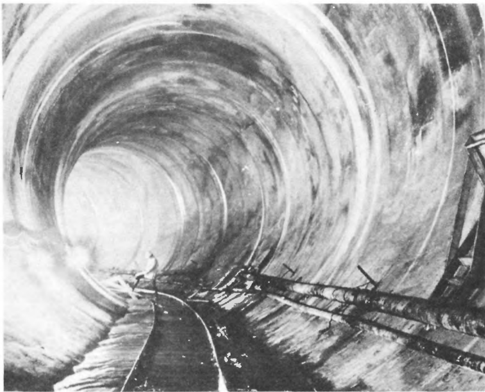
A worker inspecting a segment of New York City's Third Water Tunnel appears dwarfed by the conduit, which is 24 feet in diameter.
