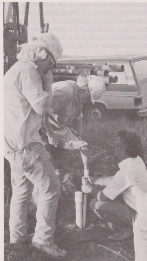
On the Fort Berthold Reservation in North Dakota, workers install a ground-water monitoring well near a dump site filled with empty pesticide containers. The Tribe has arranged for cleanup of two such dump sites, and is monitoring surface water and ground water for pesticide contamination.
