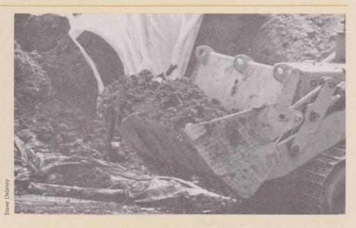
engineering activities, such as pumping and treating ground water, capping with waterproof clay, and installing drains or liners.
